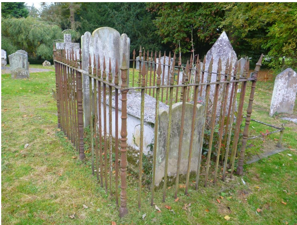
Fig. 57: Grave of John Pottrell who died in 1810, surrounded by cast iron railings that are in need of maintenance and painting.
