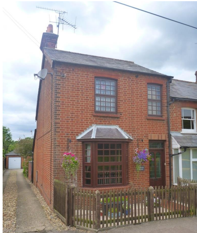
Fig. 41: Sycamore Cottage (west side) – Category 2 End of terrace house, later than its attached neighbours, and appears to date from the early-C20th. Red brick and slate roof, with a gable chimney and a ground floor bay window.
