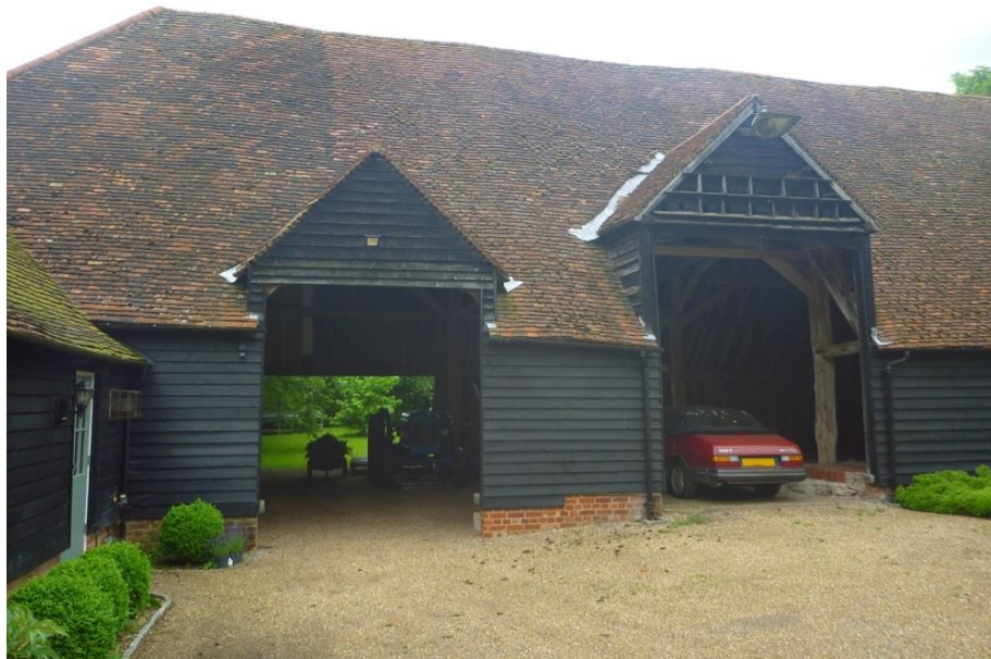
Fig. 9: Barn at Furneaux Pelham Hall
