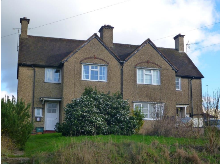
Fig. 46: 5 and 6 Lake Villas (east side) – Category 2 Two storey mid-C20th semi-detached houses with pebble-dashed render and tiled roof. Twin-gables fronting the street and arched brick detailing above the first floor windows. Three chimneys - central shared axial chimney and gable chimney each end.
