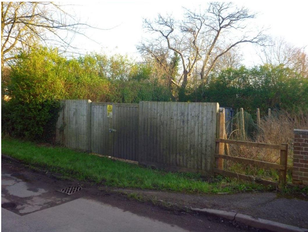
Fig. 73: The fence around the substation on The Street, just West of The Brewery Tap PH, is lacklustre in design, and the wire fencing to the side is damaged and insecure. The owner should be encouraged to enhance the site by erecting a new, more appropriate, boundary treatment.
