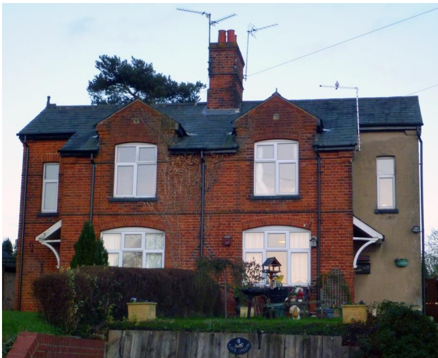
Fig. 47: 3 and 4 Lake Villas (east side) – Category 2 Two-storey late-C19th semi-detached houses. Red brick with slate roofs. Prominent central brick axial chimney stack. Two first floor windows with gablets through broken eaves to front. Cementitious render to RHS part of No 4 which has spoiled the symmetry and harmed the character of the building.
