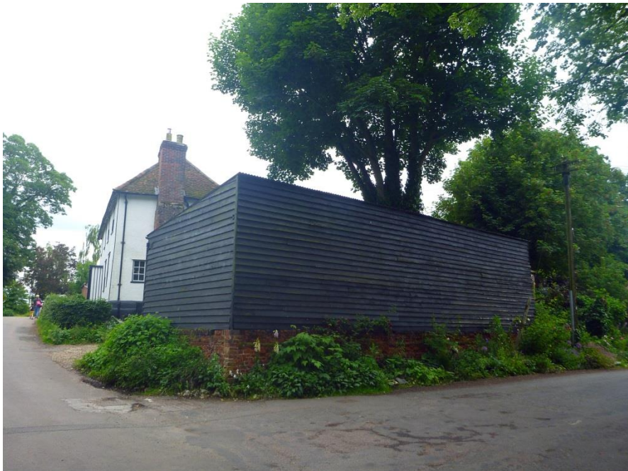
Fig. 63: This outbuilding forms a strong barrier on the corner of The Street and The Causeway. Any changes to this building should retain this character.
